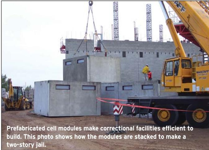
Prefabricated cell modules make correctional facilities efficient to build. This photo shows how the modules are stacked to make a two-story jail.
