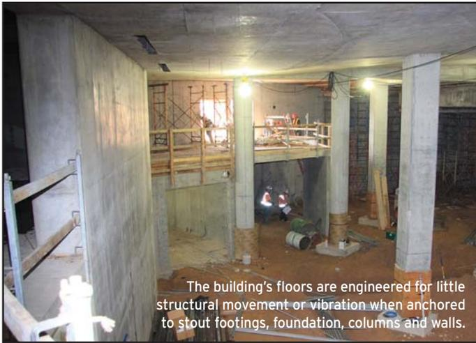
The building's floors are engineered for little structural movement or vibration when anchored to stout footings, foundation, columns and walls.
